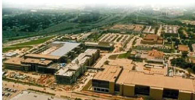
Texas Instruments will gradually invest more than $3 billion in a new 300-mm. silicon wafer fabrication facility north of Dallas – part of a global wave of new investment and reinvestment in the sector.
